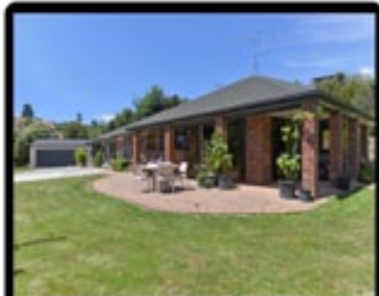
22 TOTARA VIEW ROAD 4 bedrooms, 2 living on 6000m 2
