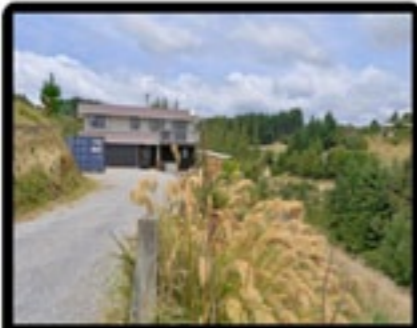
31 TOTARA VIEW ROAD 3 bedrooms on 7351m 2
