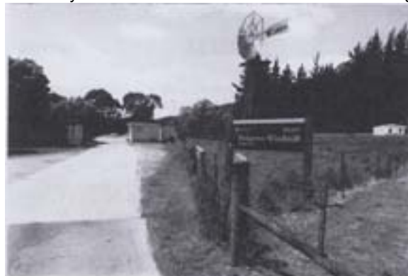
The bats show the site of the Belgrove Station and PO., now a road vehicle weigh station. The windmill, preserved, is on the right. Photo by Roger Batt 2014
