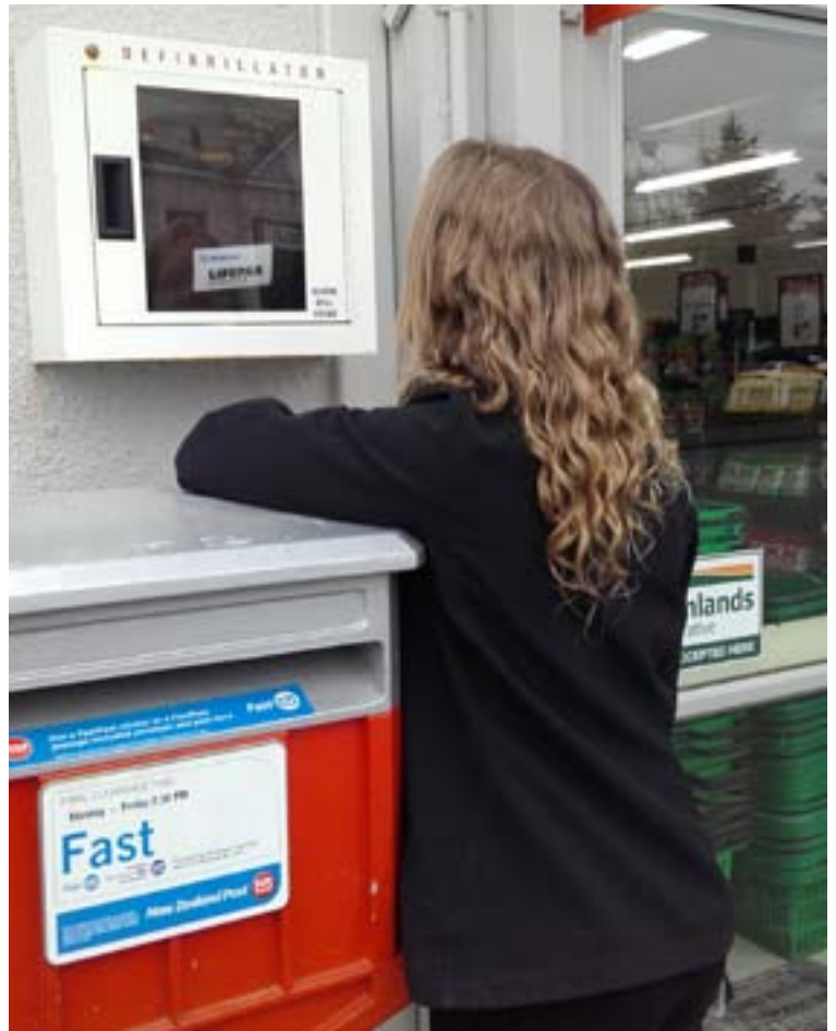
The battery has already been replaced since it was installed.
