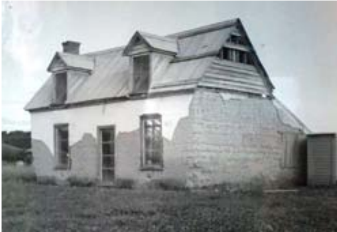
The William Higgins Gallery built in the second half of 1842 before restoration. Courtesy Cathy Cambridge. Perhaps the oldest cob cottage in NZ still in current use as a dwelling.
